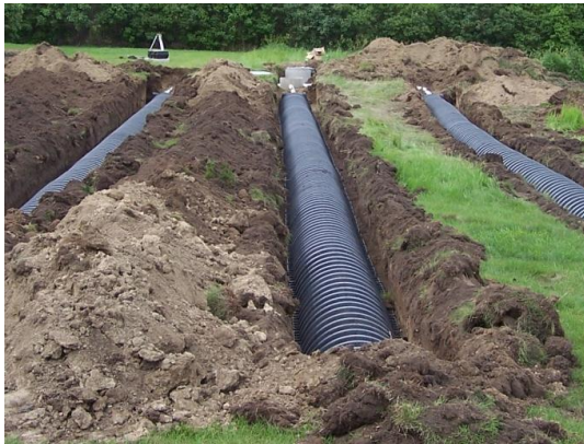
The Chamber Trench
