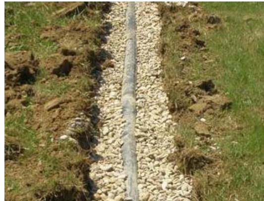
The Rock and pipe Trench
